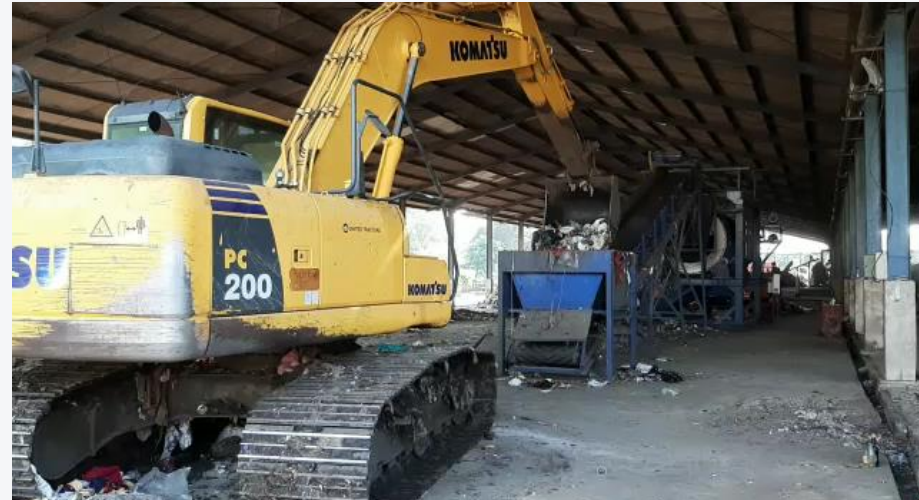
Feeding sampah ke hopper conveyor
